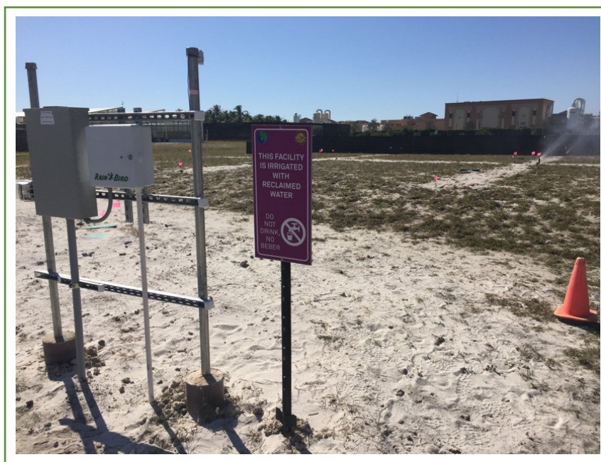
Picture 2. Freshly sprigged Celebration bermudagrass on newly constructed irrigation system. Picture taken February 5, 2020.
